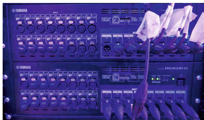
Yamaha Rio1608 stageboxes are connected to the Yamaha CL consoles over the Dante network
