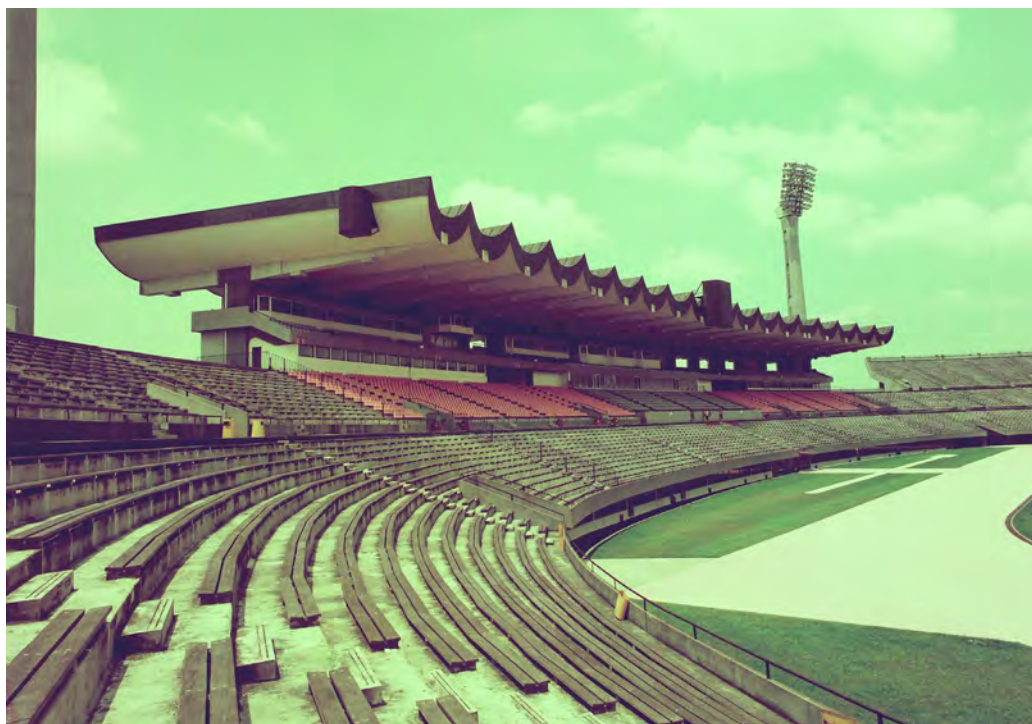
The old National Stadium that featured Altec Lansing loudspeakers installed by E&E.
