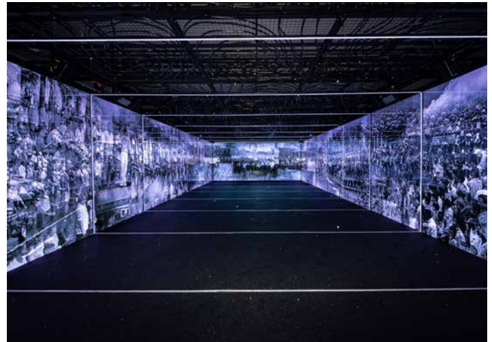
Act 5 where "rain" showers down at the guests. The top features tubes that carry the water. The flooring allows the water to flow through to a catchment underneath that recycles the water. The LED screens are protected from the water with a glass front.
