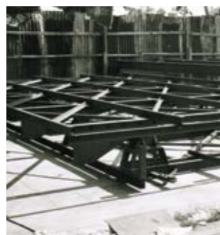
Fabrication of an extendable stage (1970)
