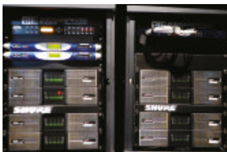
Powersoft K3 and Ottocanali 12K4 amplifiers power the EAW systems in the main sanctuary and baptismal hall, respectively
