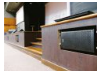
Six EAW JF8 speakers serve as front-fills built into the lip of the stage
