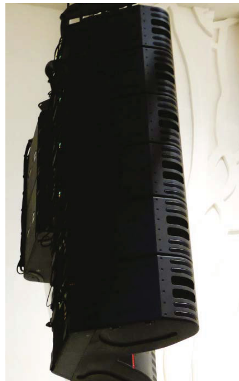
The L-R FOH system in the main theatre consists of eight-per-side Anya modules supplemented by four Otto sub modules on an adjacent hang
