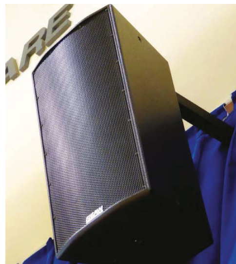
One of the MK2396i cabinets suspended in a L-C-R configuration as the main FOH system
