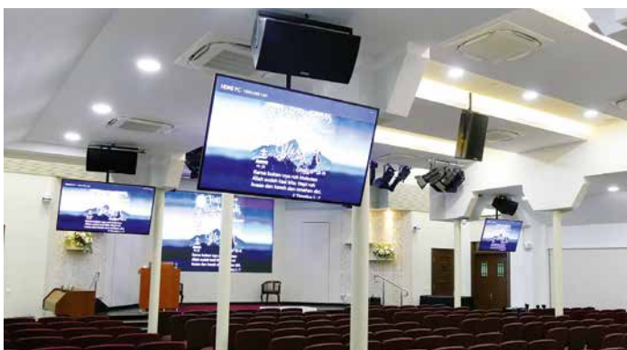
The main sanctuary is equipped with a distributed EAW MK5396i and MK2396i speaker system
